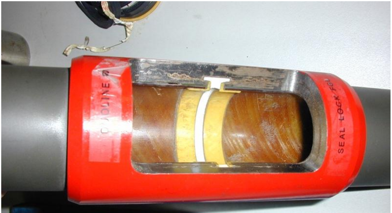
Seal at connection – teflon insert.
